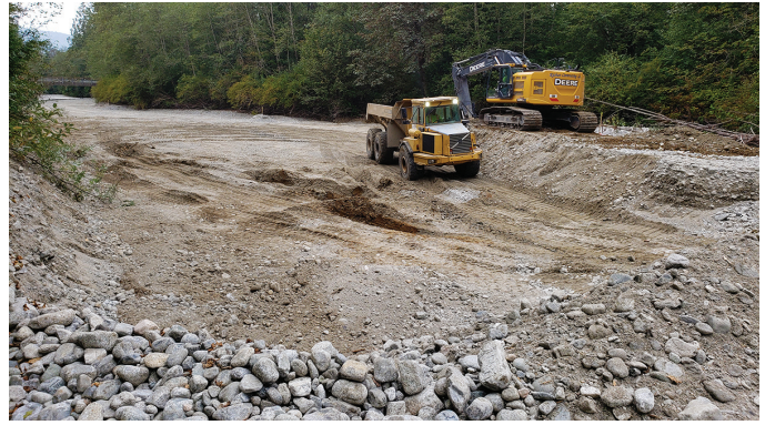
Crews removed a large amount of debris from Cascade Creek that was deposited during the 2021 atmospheric rivers.
